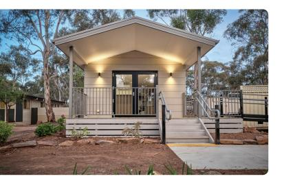
Each cabin offers two bedrooms, a kitchenette, a living area, and a veranda, while the park office supports reception and management operations. Built using volumetric modular construction, the project minimized on-site disruption, integrated energy-efficient systems, and provided high-quality, cost-effective facilities to boost regional tourism and enhance guest experiences.
