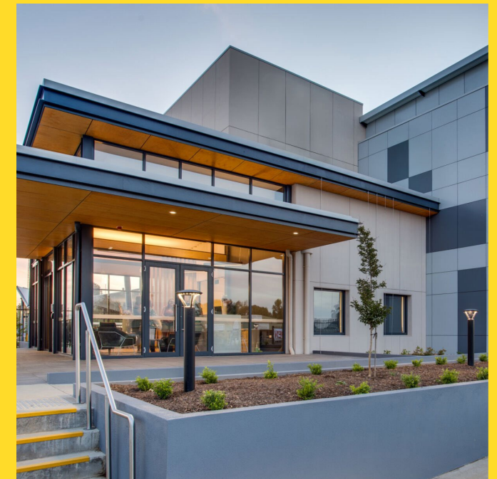
Modern workforce accommodation BOO(T)
