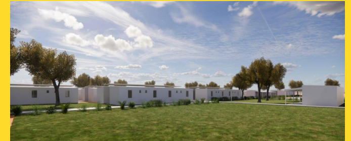
Traditional workforce accommodation
